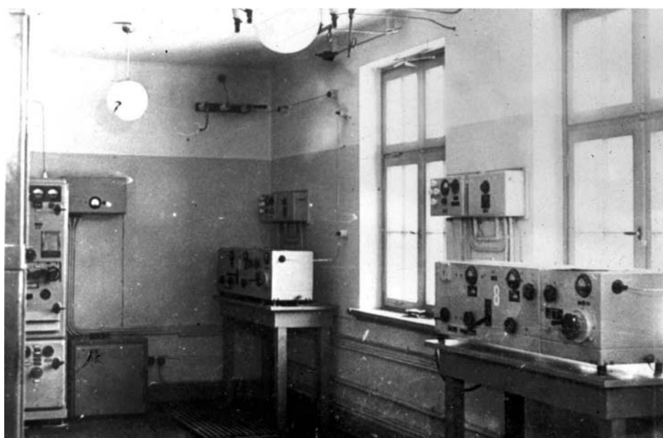
Figure 7 Adjacent to the windows, we see two Lorenz transmitters type Lo 150 FK 38. The designation FK stands for “Fern-Kurz” (short-long). The German Navy distinguished between short waves (in respect to communication distance), with an upper frequency at
